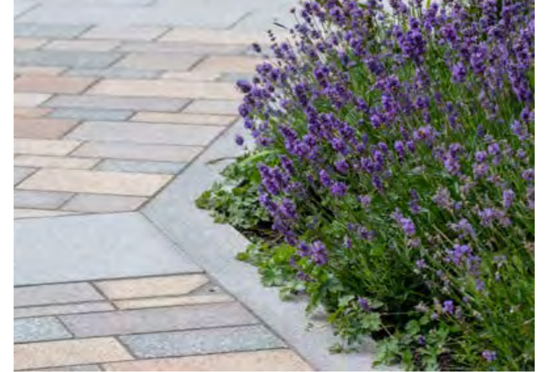
Image 2 | The public realm design will use high quality materials to integrate with the award winning University of Glasgow Western Campus
