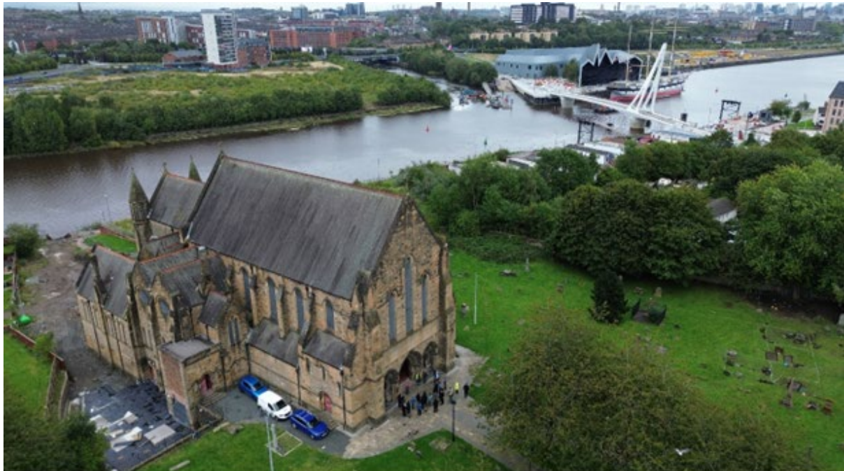
Aerial view of Govan Old showing the new bridge. (Image: R. Ferro).
